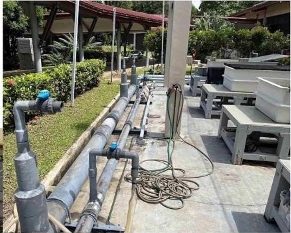
Outdoor benches with filtered light & continuous sea water supply
