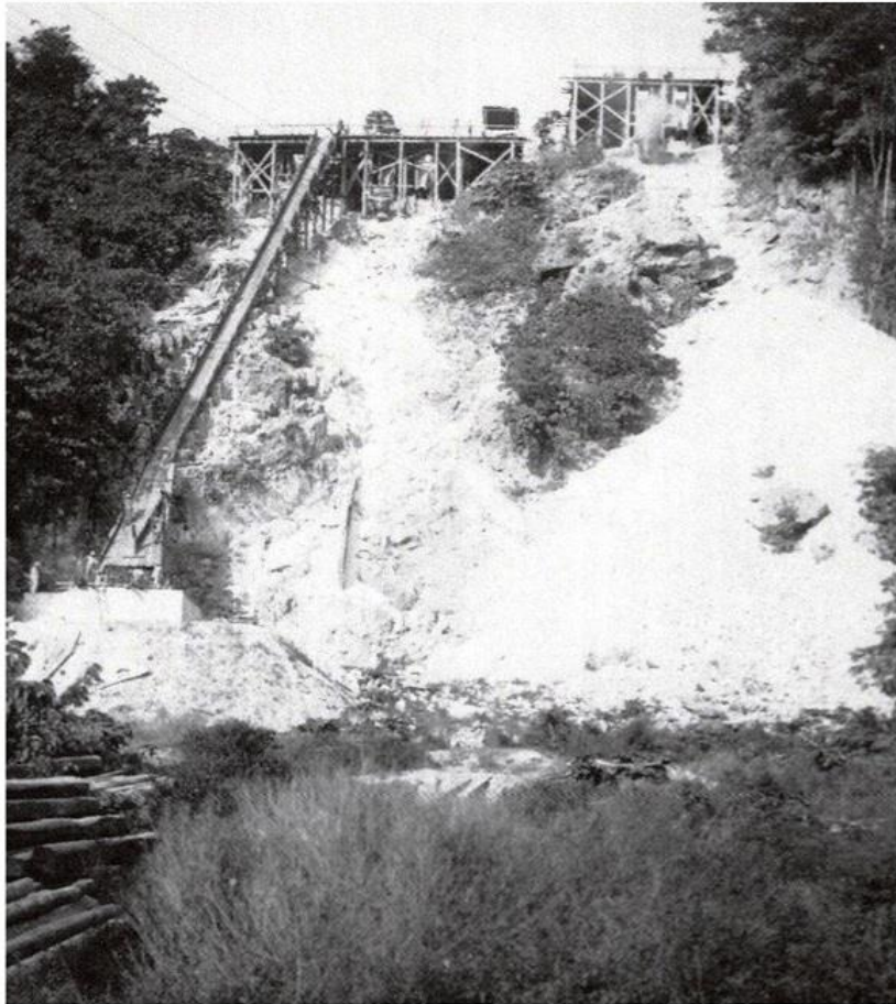
The gravity chutes, taken on the 12 September 1911 with the original tip-head chute on the right and its upgraded replacement on the left with the stone landing located in the vicinity of today's roundabout. The chutes were abandoned with the opening of the incline in 1915. Collection of the National Archives of Australia (NAA R32/16 CIPC 3)
