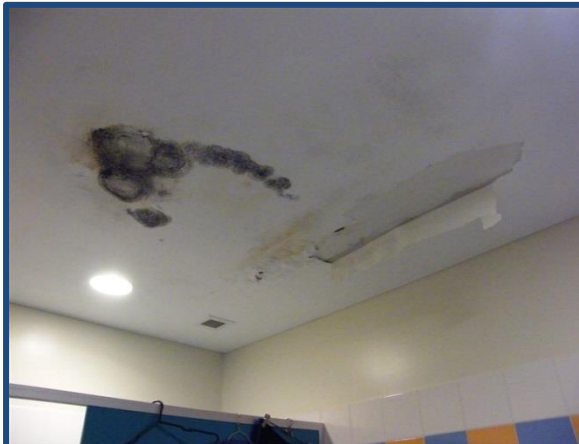
Rec Centre Male toilet - water damage to ceiling
