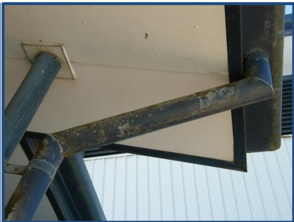
Rec Centre Air condition units, gutters, down pipes and flashing showing signs of deterioration
