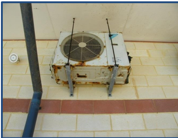
Rec Centre Air condition units, gutters, down pipes and flashing showing signs of deterioration
