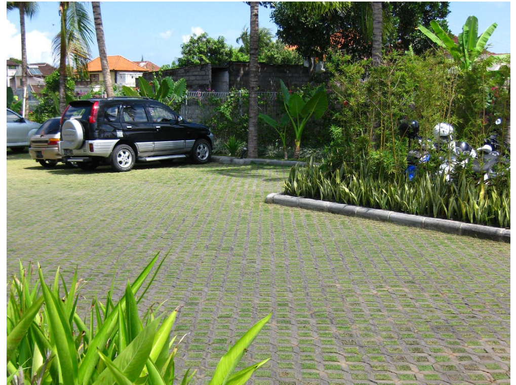
Permeable paving will provide an additional green space as well as reducing stormwater runoff from road surfaces
