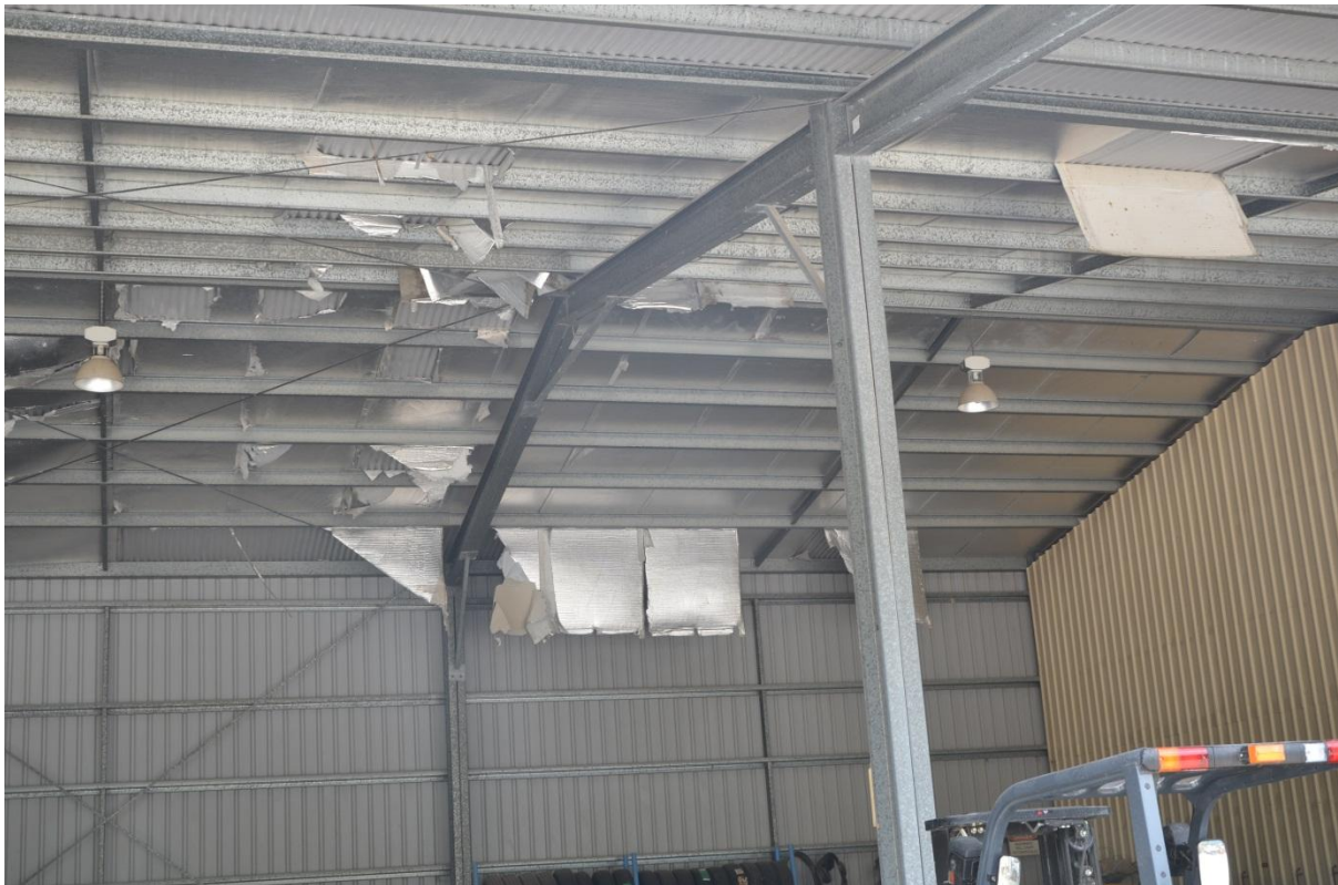
Figure 3 - Damage to Council Depot Roof Lining, Oct 2012
