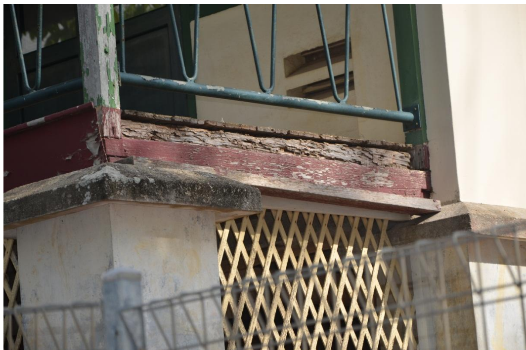
Figure 6 - Timber decay, George Fam Administration Centre, Oct 2012
