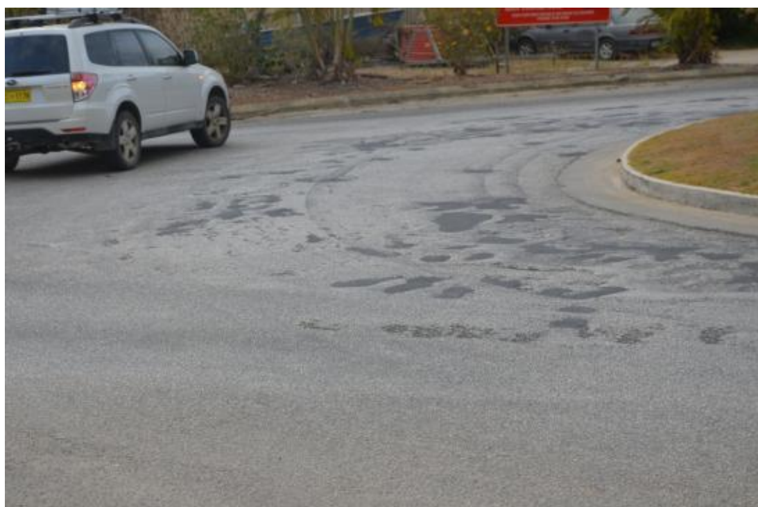
Seal slippage and patching at roundabout (Oct 2012)
